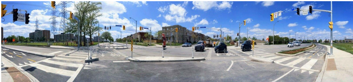
Toronto's first protected intersection at York University, featuring corner islands, bicycle signals, zebra crossings, shark teeth (yield markings), two-way cycle tracks and tactile walking surface indicators
