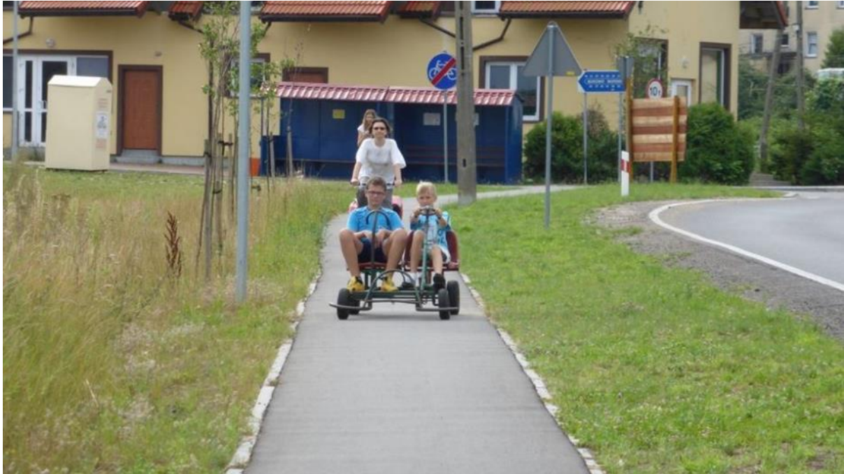
Good quality asphalt surface, but not wide enough for comfortable bidirectional traffic. EuroVelo 10.
