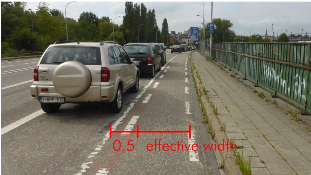
Example: effective width of a cycle lane reduced because of lack of safe distance from parked cars.
