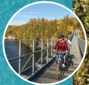
Ranney Gorge Suspension Bridge
